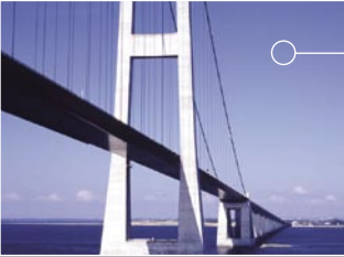
Toll collection on Great Belt Bridge in Denmark
