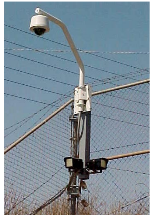
Pointed towards dark areas of sensitive locations, UF500 IR Illuminators used with PTZ domes enable effective surveillance even under night-time hours. Patent# 6158879.
